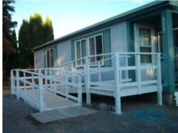
A ramp, built by InterLink in Clarkston, helps a client access her home more easily
